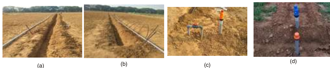
Fig.-2 : (a) Laying of main line, (b) Laying of sub-main with punched laterals, (c) Gate and air release valve,
